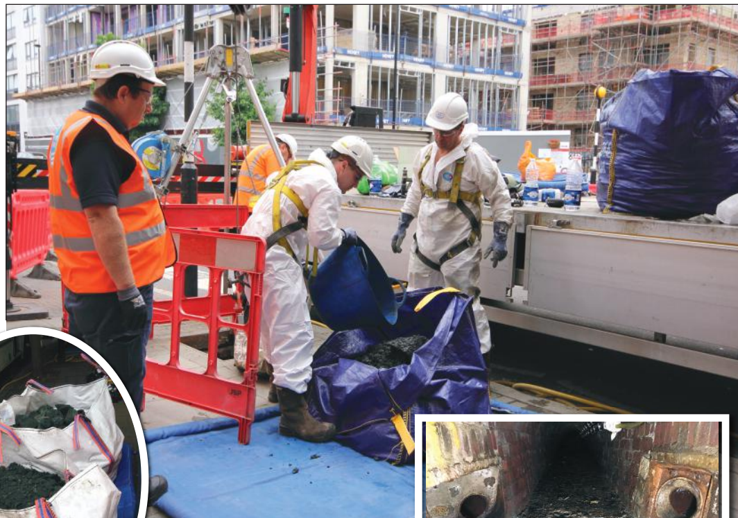
Far left: Thames Water employees work in the confined space before breaking up the concrete, above, and putting it in bags, circled left; The concreteberg in situ is seen, right
